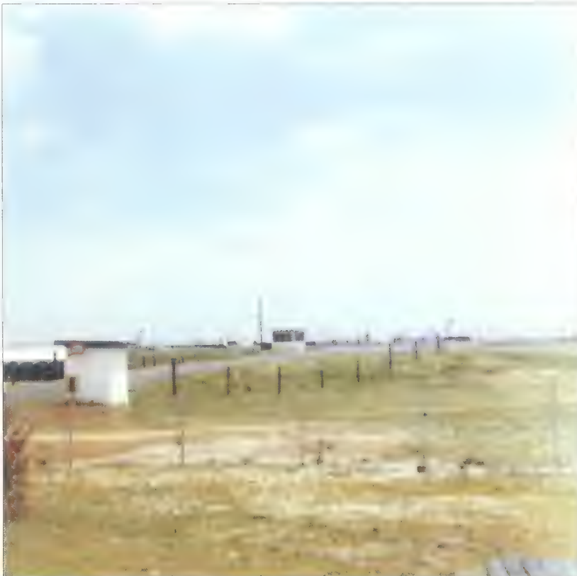
Figure 4.25. View looking northeast at the Missile Magazines, NIKÉ launch site, circa 1968. During the historic period, vegetation was maintained at the launch site and no large woody vegetation can be seen in the Missile Maintenance Area. The Paint and Oil Storage shed (447) can be seen on the left foreground (GATE 22041).
